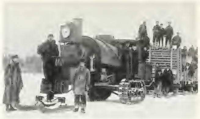
Sled traction engine pulling cord wood.
