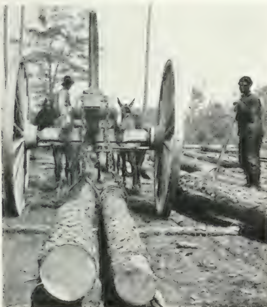
Slip-tongue arrangement of high wheeler, seen from behind.
