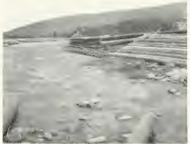
Fixtures along the banks of a stream used for splashing and driving.
