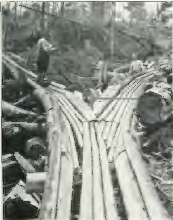
Junction of two pole chutes, holdings of Champion Lumber Co., North Carolina.
