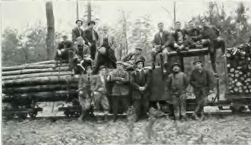
Biltmore Forest students inspecting a portable forest railroad; notice the minute trucks, and the small six horse-power gasoline motor. Darmstadt, Germany.
