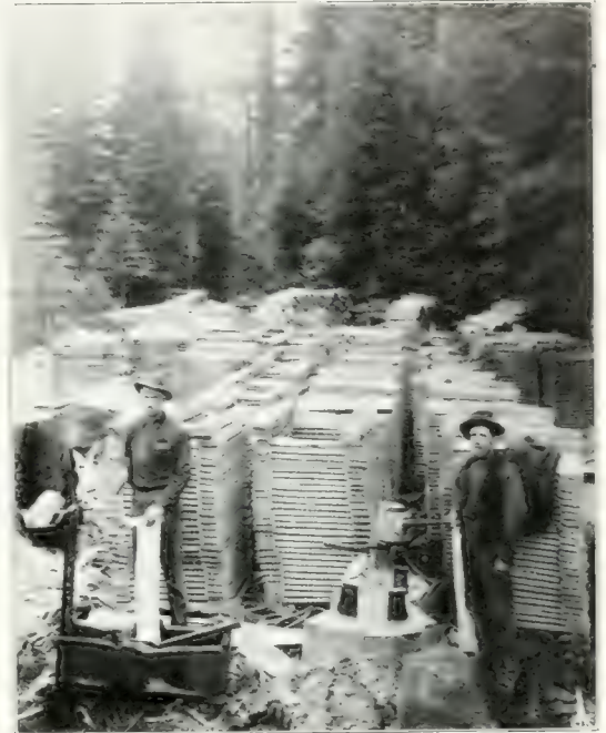
The manufacture of rived sugar pine shakes in the Sierra Nevada.
