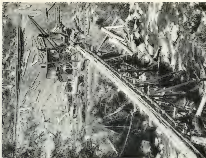
A donkey pulling a string of logs over a slide across a deep ravine in Western North Carolina; in the rear the dumping place of a log slide and a steam log loader.
