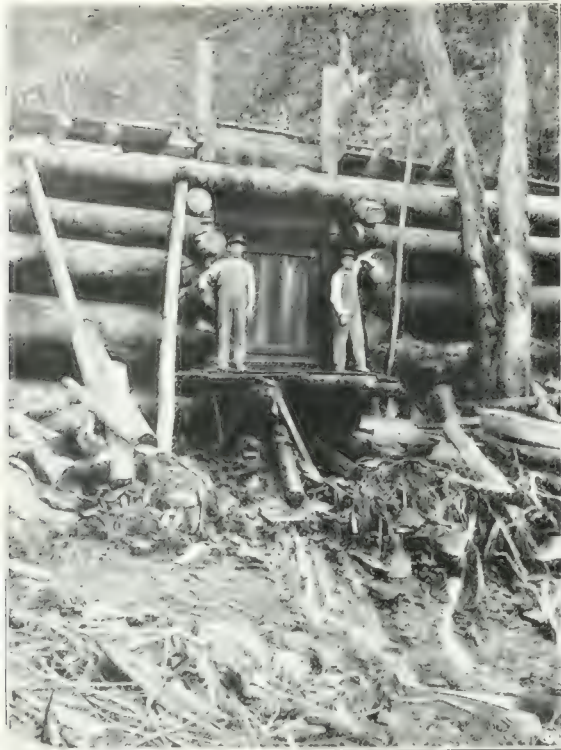
Small splash dam, seen from below, at the summer camp of the Biltmore Forest School.
