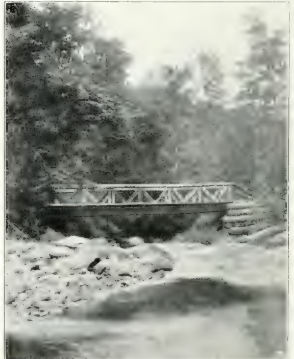
A bridge spanning 85 feet across Davidsons's River, Biltmore Estate. The two white oak cribs supporting the bridge contain each 1,500 feet b. m.
