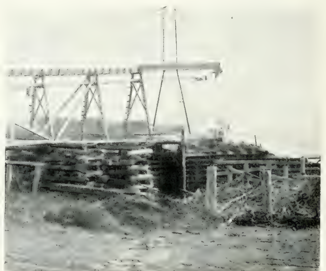
Waste conveyor and open burner at a Maine sawmill.
