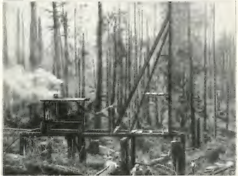
Piledriver of Smith-Powers Logging Co. at work on Coos Bay, Oregon.
