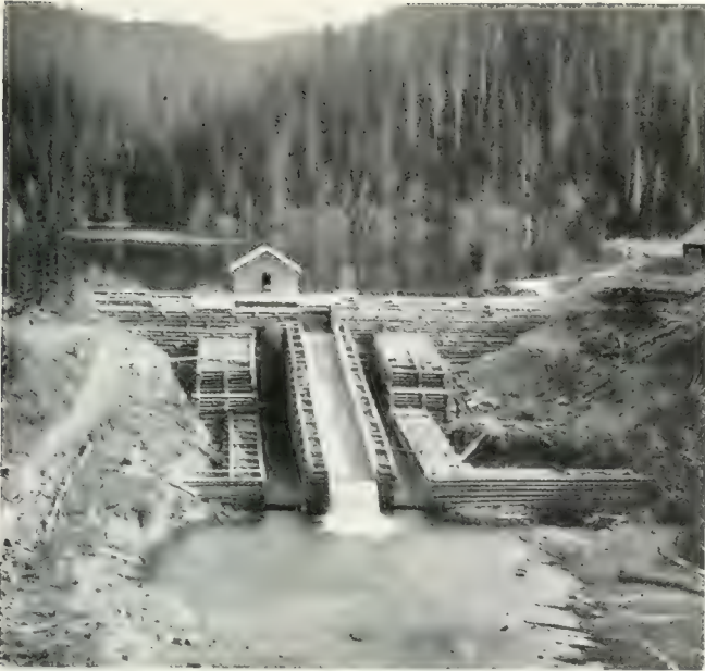
Large splash dam in the Karpathian mountains. The small ladder protruding from the top of the dam opens a small gate by which the fore-water may be given.
