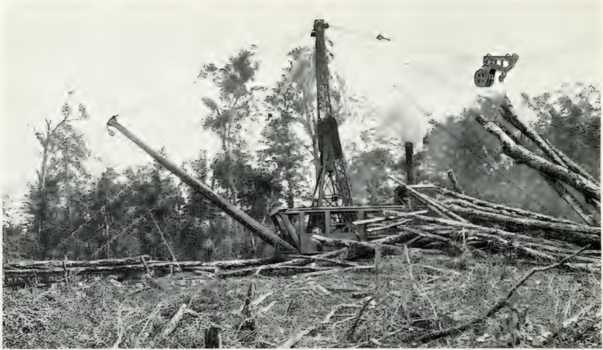
Aerial logging, with main spar at loading engine. Lidgerwood Mfg. Co., Liberty St., New York.
