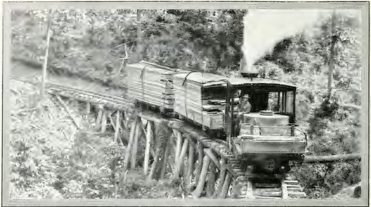
Climax engine in operation on a trestle, over wooden rail. Climax Mfg. Co, Corry, Pa.
