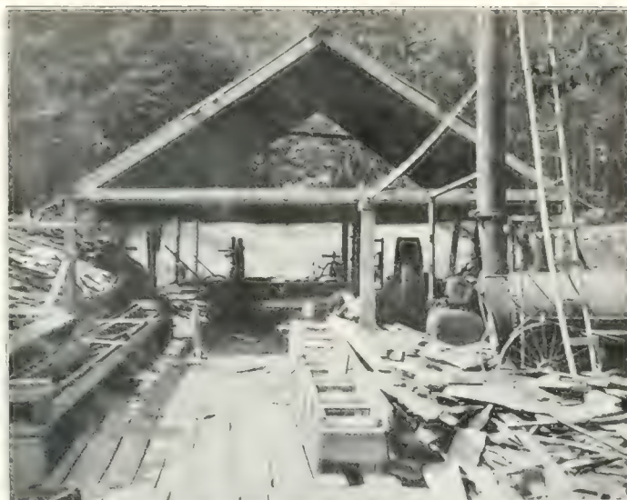
Thirty horse-power portable circular mill on Biltmore Estate, North Carolina.
