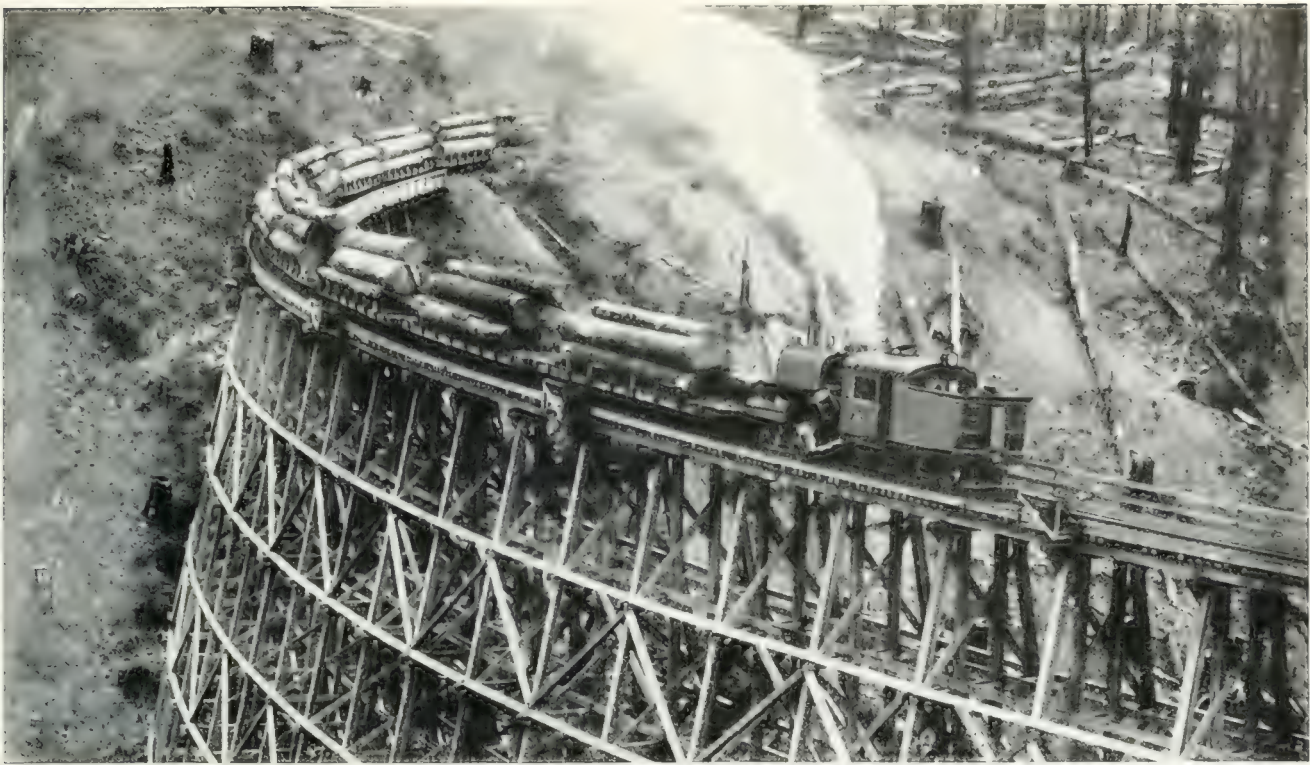
High trestle bridge and sharp curve negotiated by a log train pulled by a Heisler locomotive. Heisler Locomotive Works, Erie, Pa.
