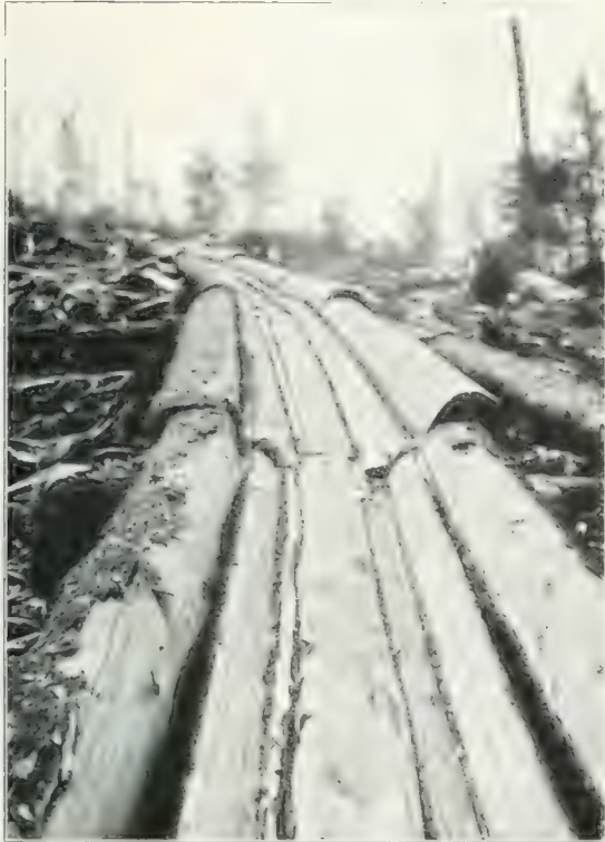
Timber chute for transportation of logs in Oregon.
