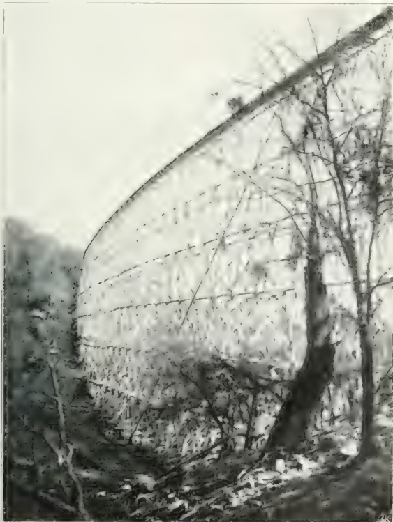
High trestle bridge carrying a timber flume in the Sierra.
