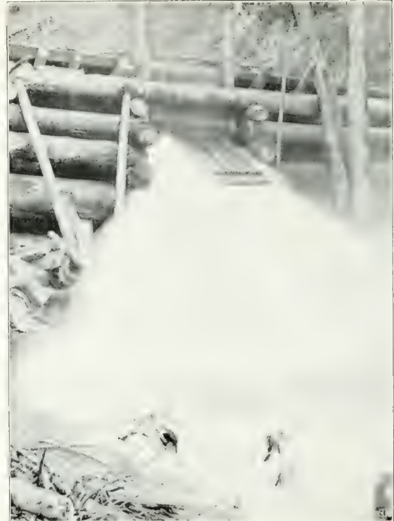
Splash dam with the gate swung open
