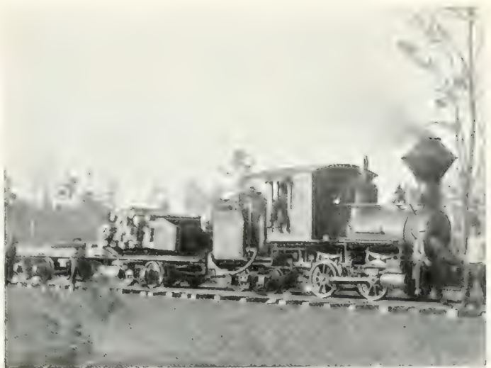
Rail-laying car and engine at work on John L. Roper Lumber Company's holdings, Eastern North Carolina.
