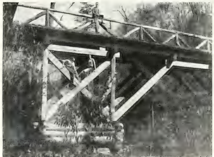
Braced bridge across Looking-glass Creek, Biltmore E state.
