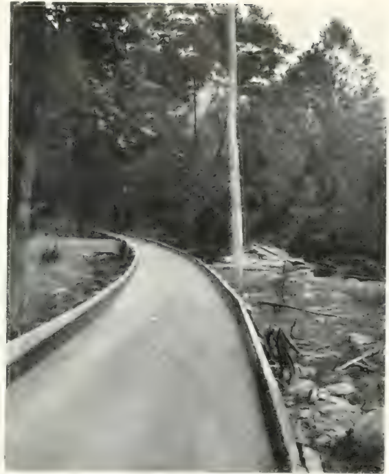
Box flume in Swaine county, North Carolina.
