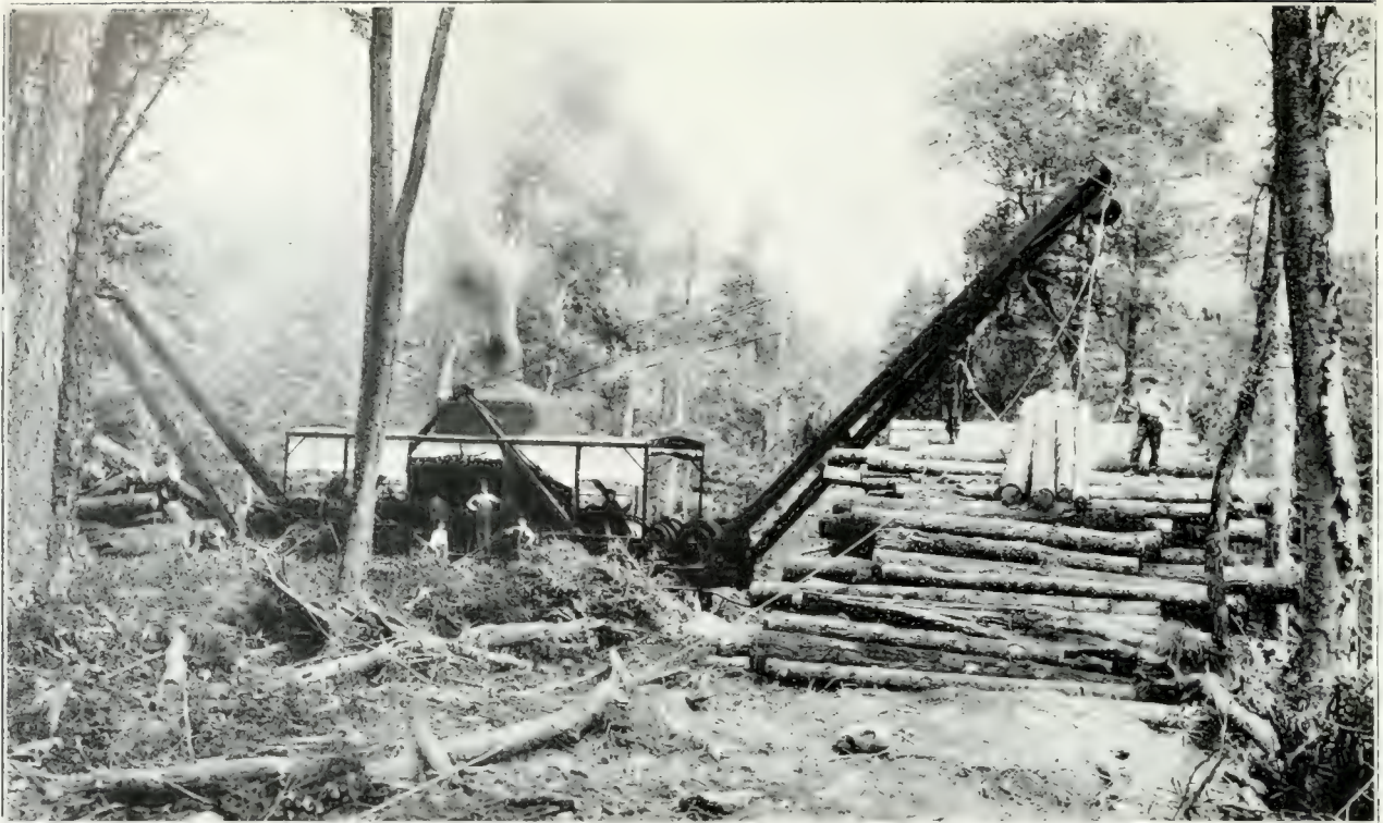
Four-line skidder in operation. Clyde Iron Works, Duluth, Minn.
