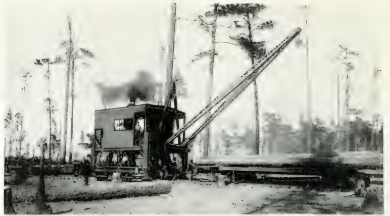
McGiffert log loader at work. Clyde Iron Works, Duluth, Minn.
